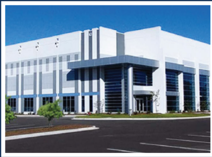
CHARLESTON TRADE CENTER Keith Corporation Summerville/Jedburg ±1,019,200 SF
