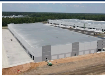
TRADE PARK EAST BLDG 1 & 3 ±516,000 SF
