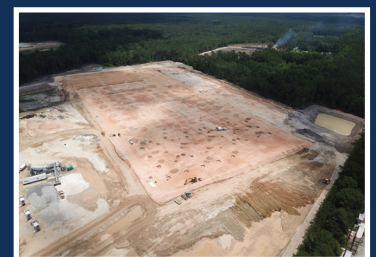
OMNI INDUSTRIAL BLDG 4 ±607,000 SF
